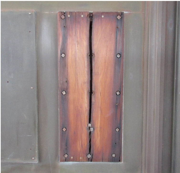
Figure 3. Original backing board on window WA5, proper lhs, segment 3/5.
