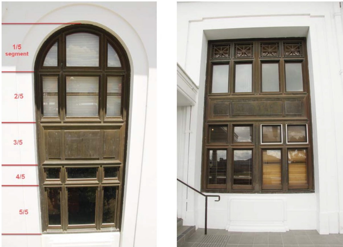
Figure 1. Nomenclature for segments of the arched and rectangular windows.
