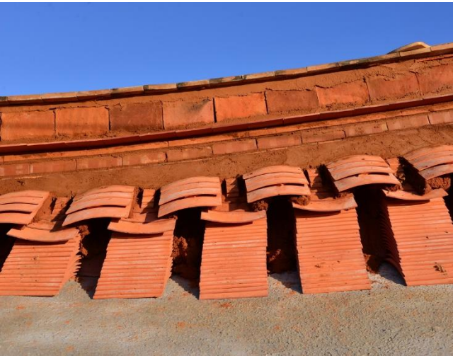
red tile roofing
