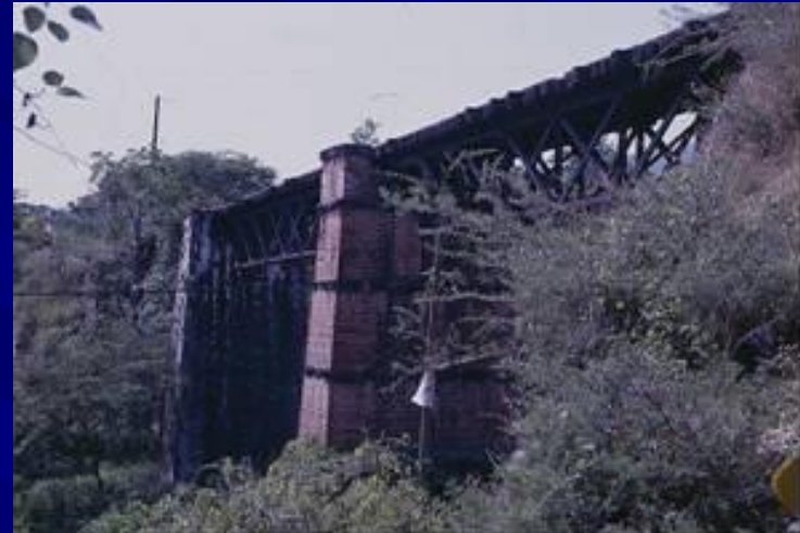
Railway bridge in Barranca Honda, Morelos. Mexico
