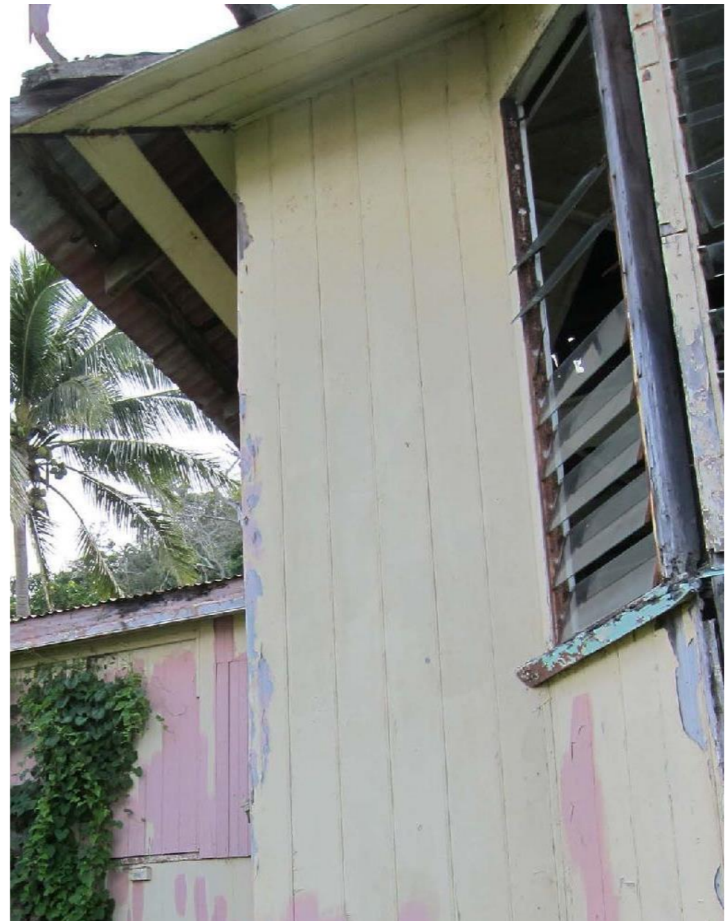
Tongue and Groove Boards
