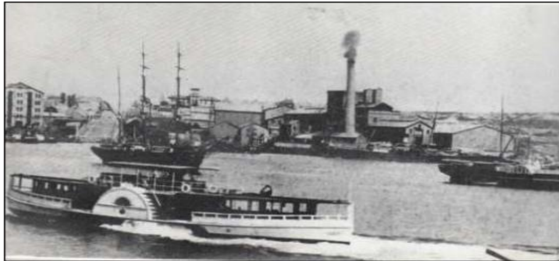
Pyrmont Sugar Refinery - 1878 Sydney Source: South Pacific Enterprises by CSR
