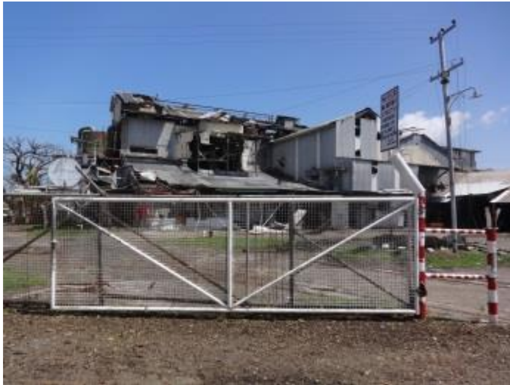
Penang Sugar Mill, post Hurricane Winston Image: Chris Richards
