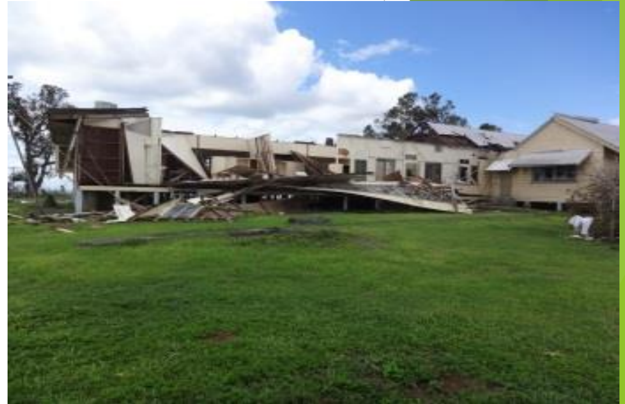
Hurricane Winston Damaged Single Officers Quarters Lautoka Sugar Mill Image: Chris Richards 2016
