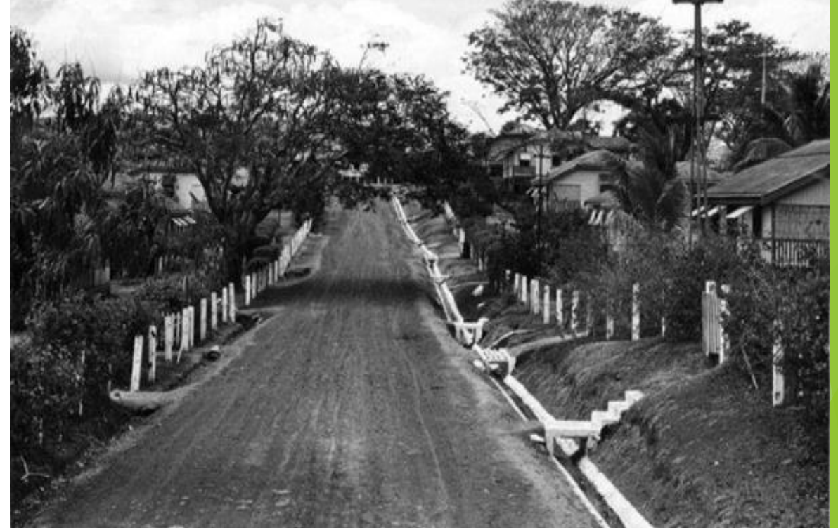
Rawari Sugar Mill Company Town Houses for Mechanics & Fitters. Circa 1950's.
