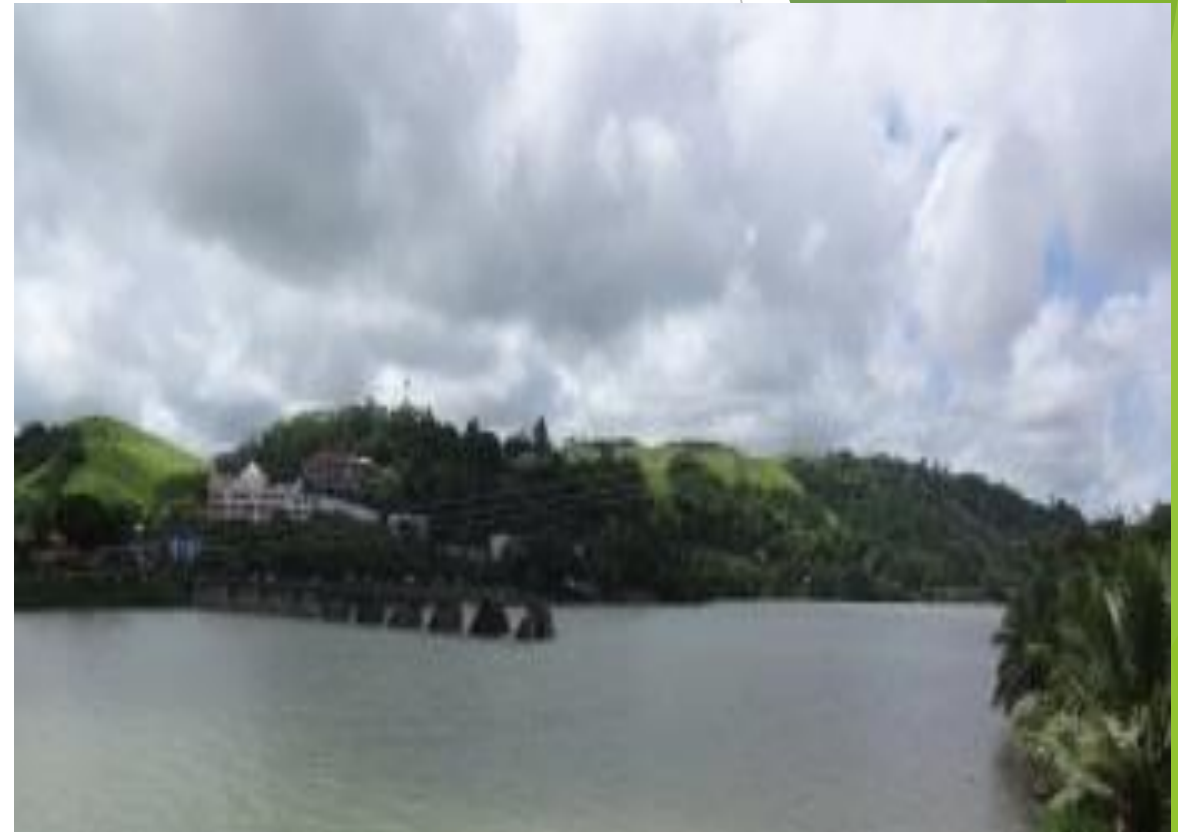
Hurricane Damaged Sigatoka Railway Bridge Image: Chris Richards 2016
