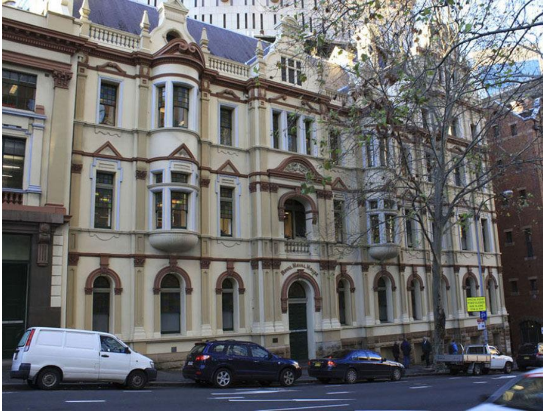
Royal Naval House ("Goodenough House"), The Rocks
